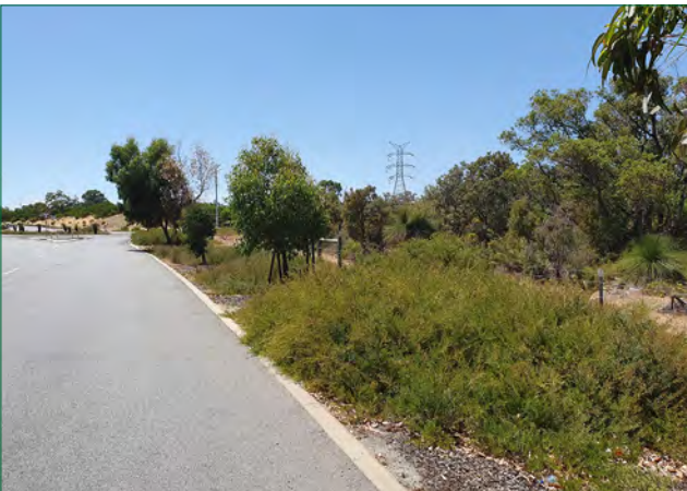
Example of vegetated roadside swale (Flinders Valley Estate, Hope Valley)
