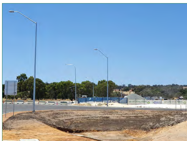
Subdivision and road works in Precinct 1A – North A
