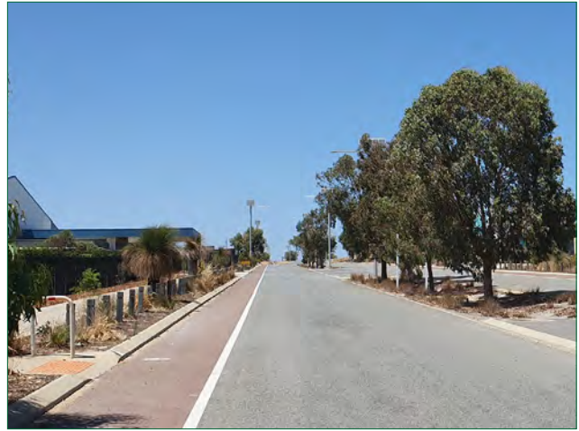
Example of landscaping along a road reserve (Flinders Valley Estate, Hope Valley)
