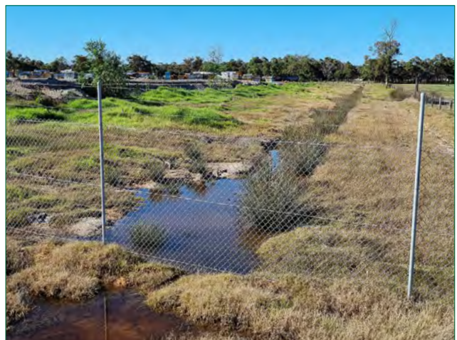
Drainage line through Precinct 3
