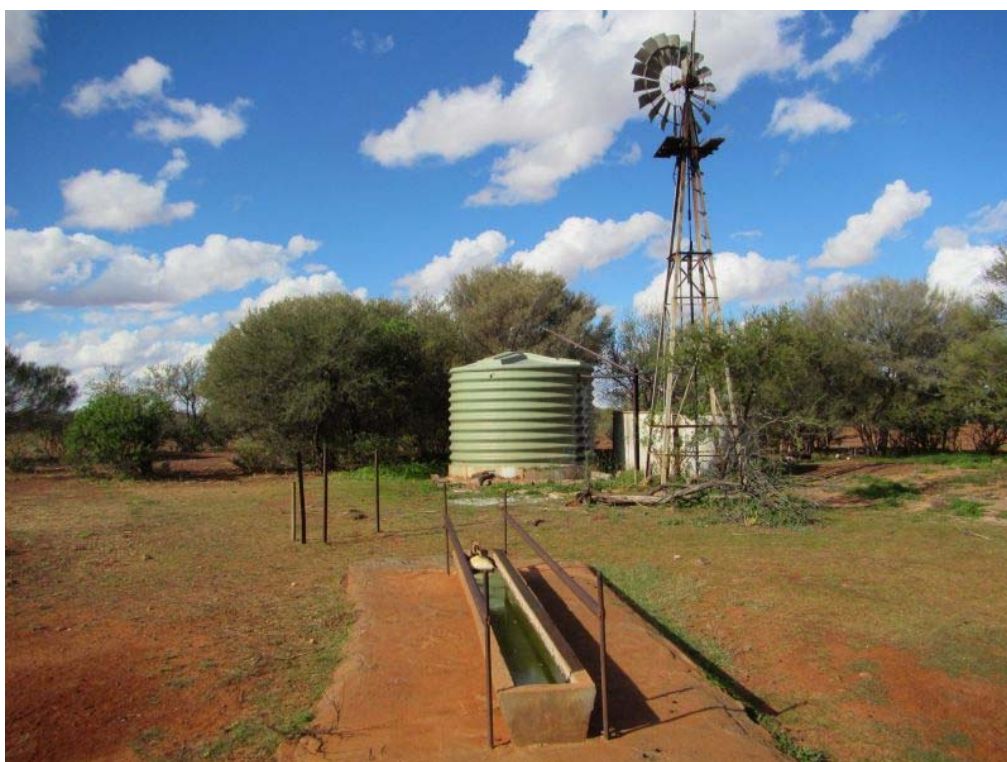
Figure C6 Stock watering trough and windmill within the Mount Magnet Water Reserve
