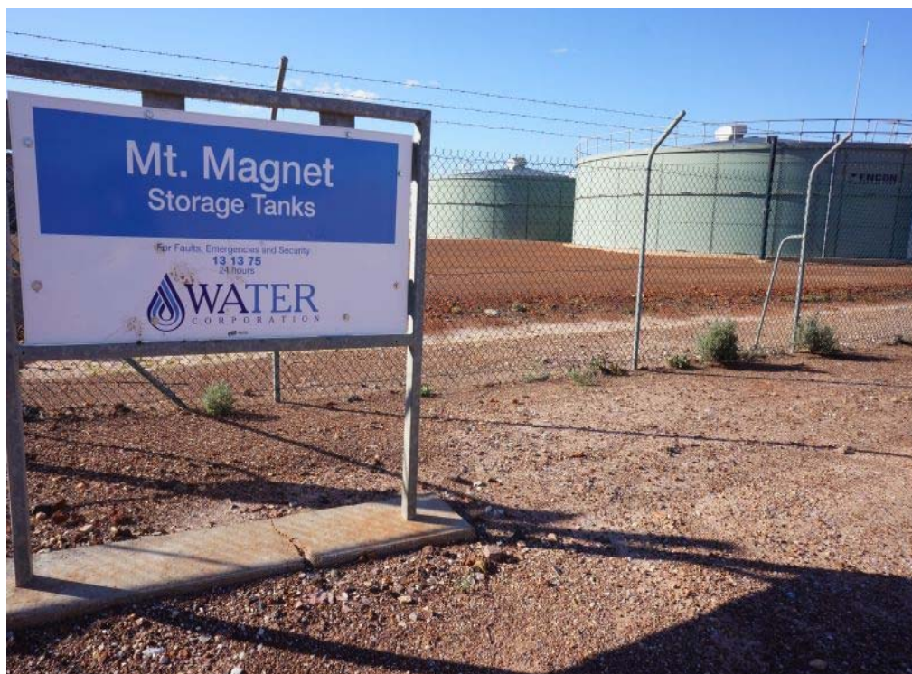
Figure C3 Mount Magnet water storage tanks
