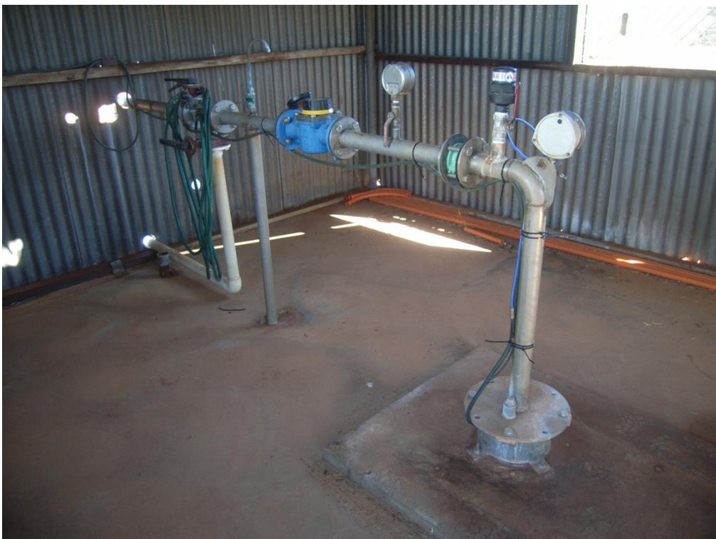
*Figure D2 Sealed production bore inside shed (Photo: J. King)*
