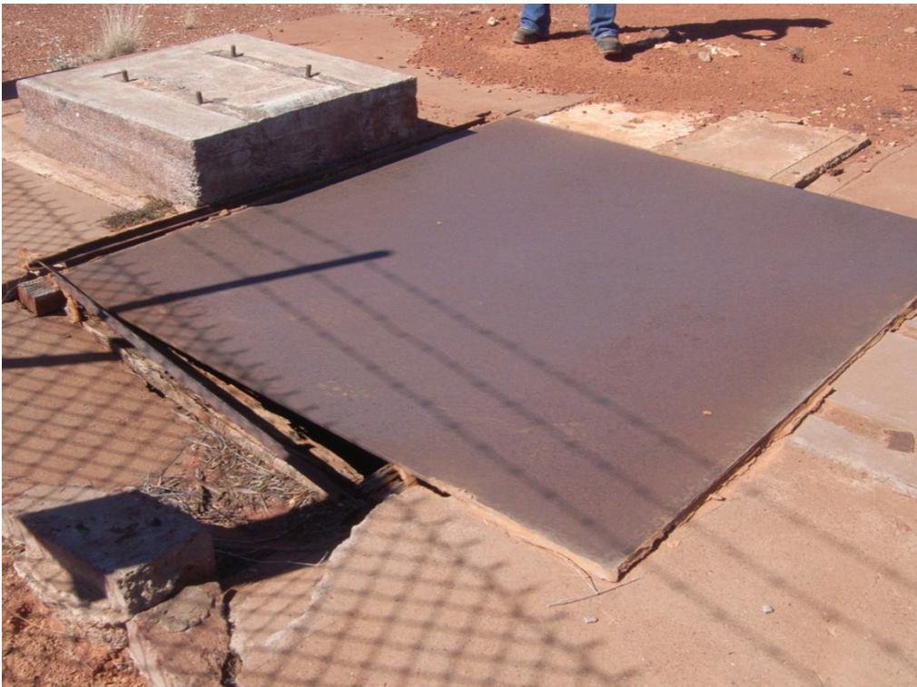
**Figure D6** Historic well within bore compound with damaged capping and seals (Photo: J. King)
