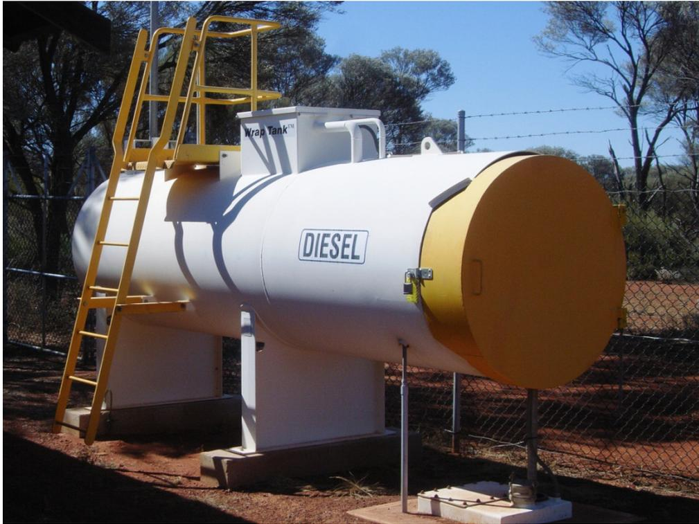
Figure D3 Self-bunded fuel storage tank with anti-theft device (Photo: J. King)
