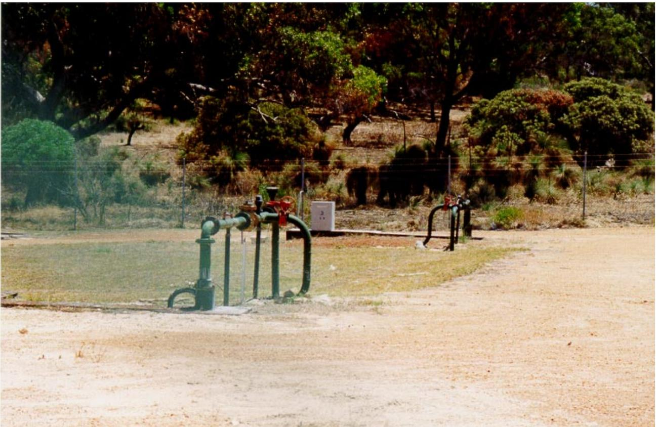
**Plate 1: Wellfield at Guilderton with bores 1/65, 2/65 and 3/69 and located in area of coastal scrub vegetation.**
