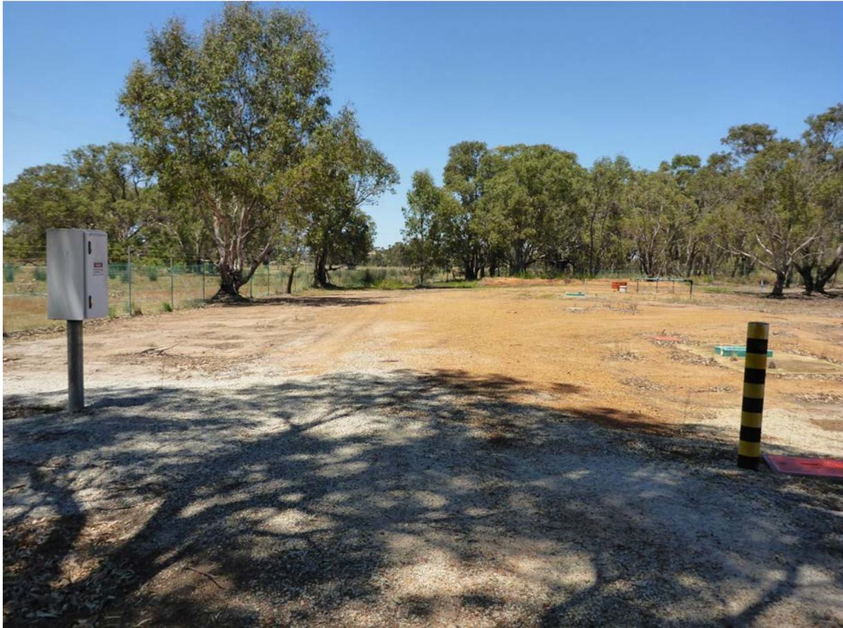
*Figure C5 Dandaragan Water Reserve – monitoring bore 2/77 on the right and failed production bore 1/82 retained as a monitoring bore in the background*
