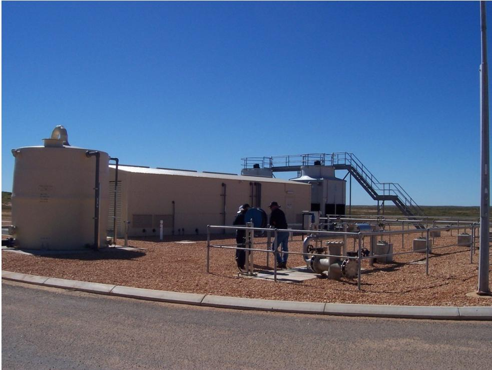
Figure D1 Coral Bay desalination plant, deep artesian bore 1/04 and cooling towers (back) [Photo: B. Franke]
