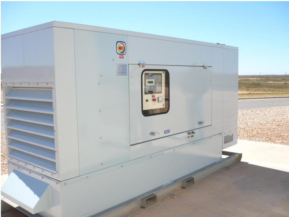
*Figure D4 Coral Bay water supply plant back-up diesel generator (self-bunded) [Photo: B. Franke]*
