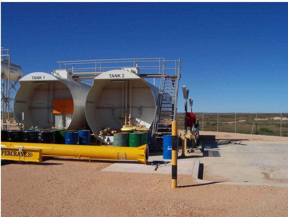
**Figure D6** Diesel storage tanks (externally banded) at the Coral Bay power station [Photo: B. Franke]
