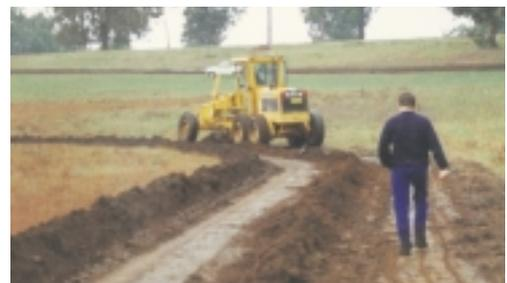
*Permanent grade banks – planned, surveyed and shown being constructed by a road grader.*
