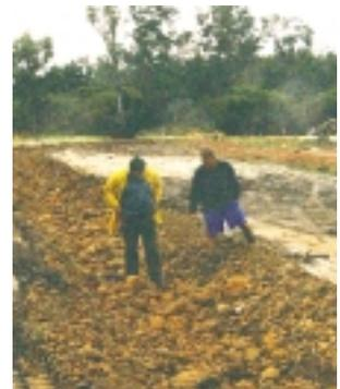
*Rocked chute under construction on an eroding sandy gully, Manjimup.*
