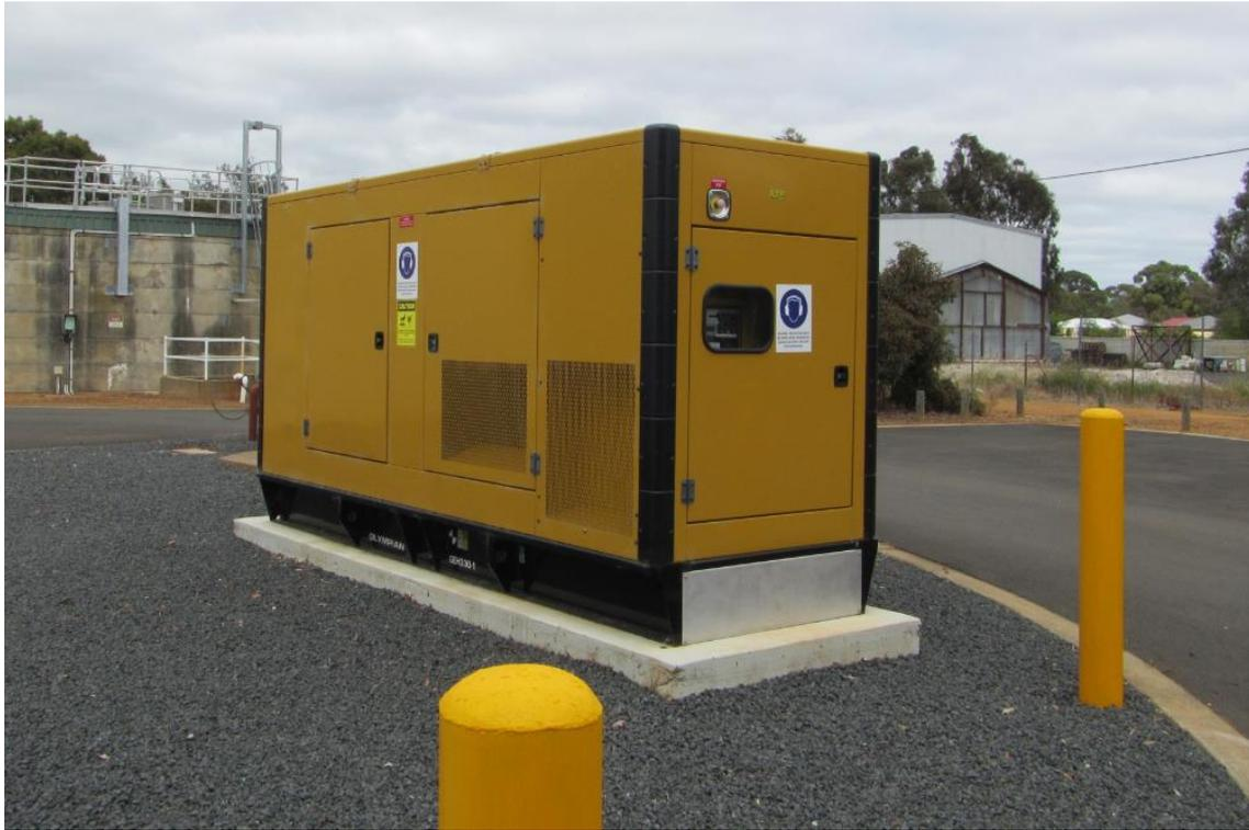
Figure D5 Self-bunded diesel generator
