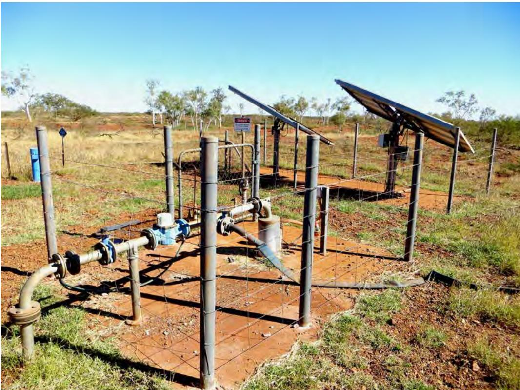
*Figure C6 A solar powered production bore within the Cane River Water Reserve, photograph by V. Cloughton, Department of Water*
