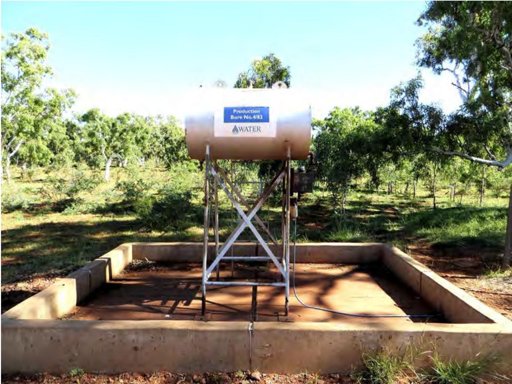
*Figure C5 A bunded fuel tank used to power a production bore within the Cane River Water Reserve, photograph by V. Cloughton, Department of Water*
