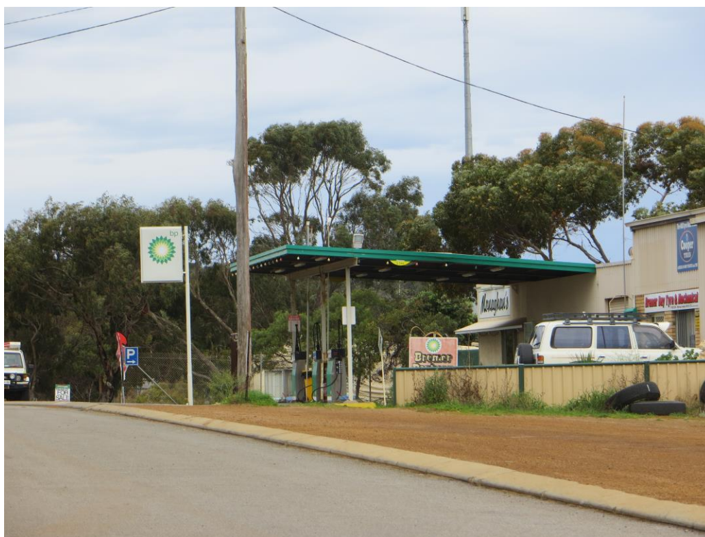
Figure D4 Service station in Bremer Bay Water Reserve
