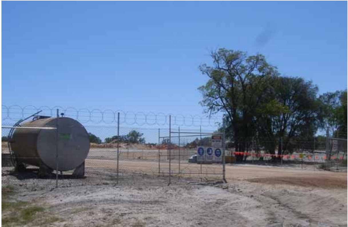
Figure C7 Picton Water Reserve drinking water treatment plant and compound under construction
