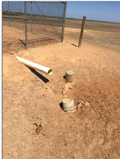
*Photo C4 Unsealed bores in Mount Hill bore field*
