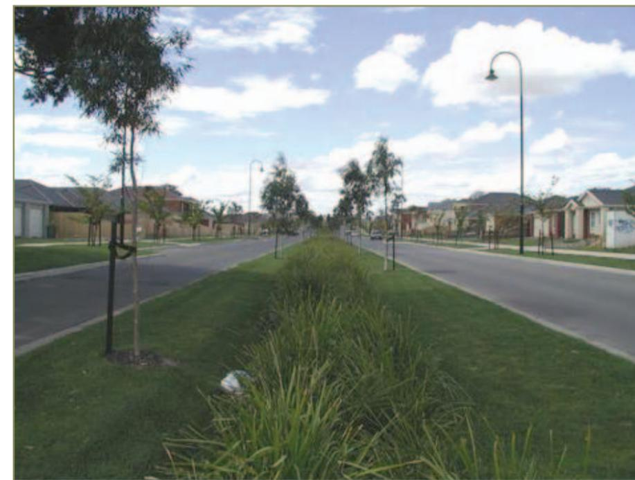
*Linear bioretention swale in multiple use corridor*
