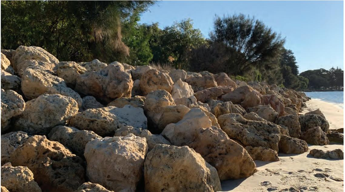
Image 16. Example of rock revetment coastal protection works.
