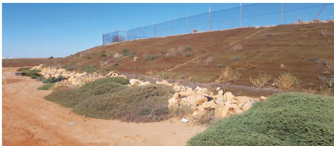
Image 15. View of the Cooke Point Road wastewater pumping station eastern boundary showing an example of 'soft edge' coastal protection using geotextile matting over sand bund with rock scour protection at the base.
