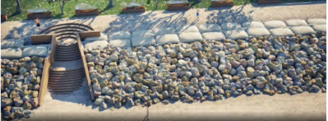
Image 20. Example of stairs integrated with coastal protection works to allow pedestrian access and connectivity with the foreshore area. (Source: Fraser Chronicle, 2020)
