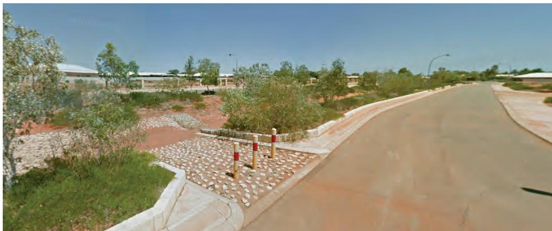
Image 23. Example in Gannet Street, South Hedland of rock pitching and kerb break to allow stormwater to discharge from road into the roadside open drain. (Source: Google maps street view, 2020)
