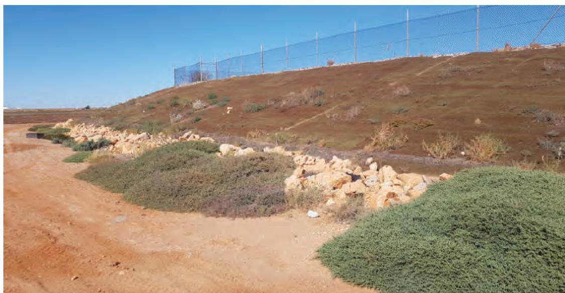
Image 18. View of wastewater pumping station eastern boundary showing an example of 'soft edge' coastal protection using geotextile matting over sand bund with rock scour protection at the base.
