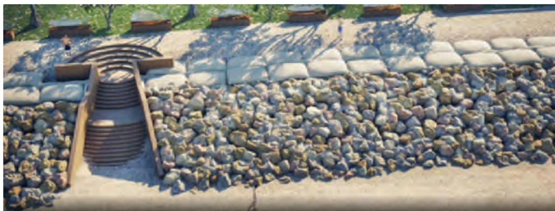
Image 26. Example of stairs integrated with coastal protection works to allow pedestrian access and connectivity with the foreshore area. (Source: Fraser Chronicle, 2020)
