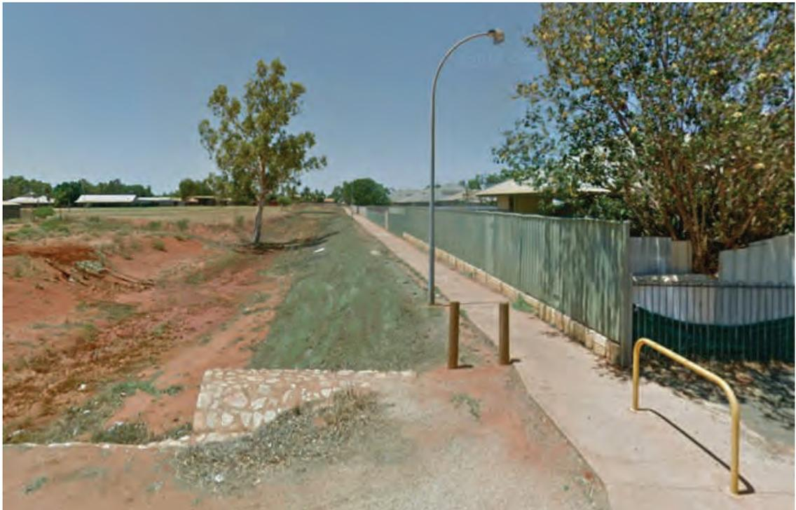
Image 29. Example in Kennedy Street, South Hedland of an open swale drain adjacent to residential lots with a side pathway. This principle is envisaged for the drainage corridors in the structure plan where provision of a pathway is considered appropriate, to increase pedestrian connectivity and accessibility to the foreshore. (Source: Google maps street view, 2020)
