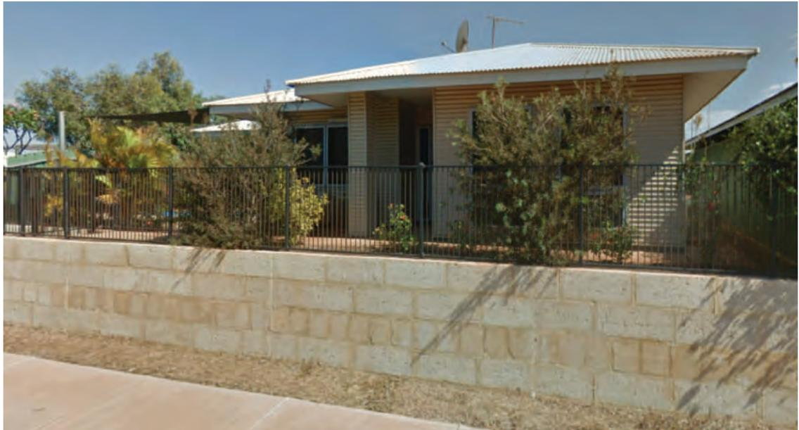
Image 25. Residential development near the intersection of McGregor Street/Cooke Point Road with visually permeable developer uniform fencing on top of the retaining wall. The site has been raised to address coastal hazard flood inundation. The proposed structure plan development interface with Cooke Point Road will likely take on a similar form as this existing development. (Source: Google maps, 2020)
