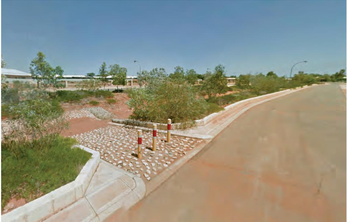
Image 28. Example in Gannet Street, South Hedland of rock pitching and kerb break to allow stormwater to discharge from road into the roadside open drain.(Source: Google maps street view, 2020)
