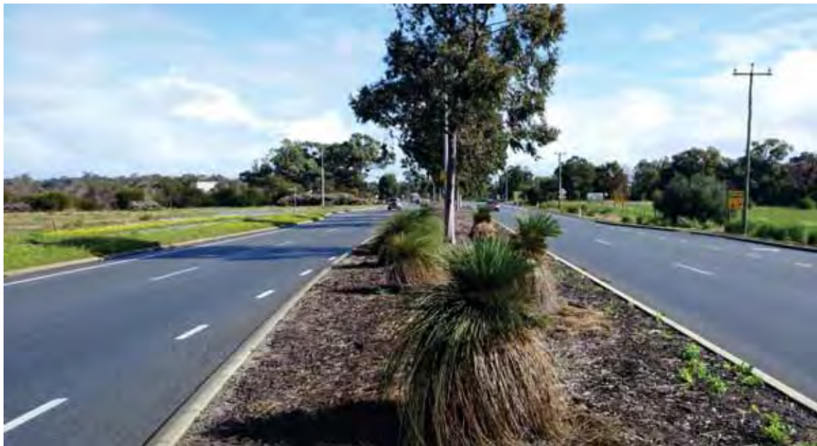
Figure 4: Westbound view along Beeliar Drive in the vicinity of LSP
