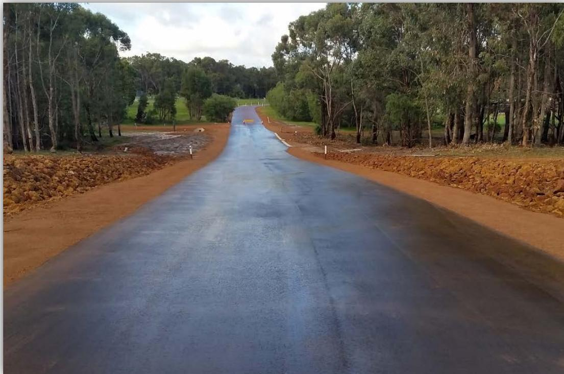
**Figure 3 - Typical Rural Formation roadway with Scour Protection and Lowpoint Kerbing**
