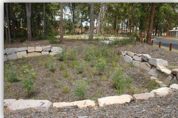
**Typical sub catchment scale bioretention basin**
