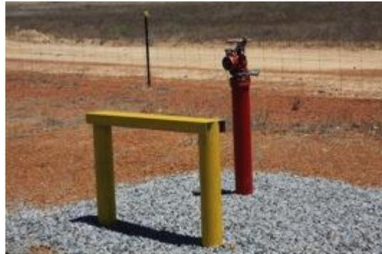
Figure 13 & 14: Example infrastructure including a 50,000 litre concrete water tank clearly identified for emergency use only (left) with the Milcock hydrant located downslope adjacent to a public road (right)
