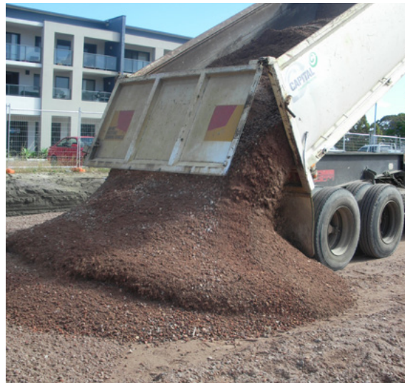
C&D waste is used as road base (© Main Roads WA)
