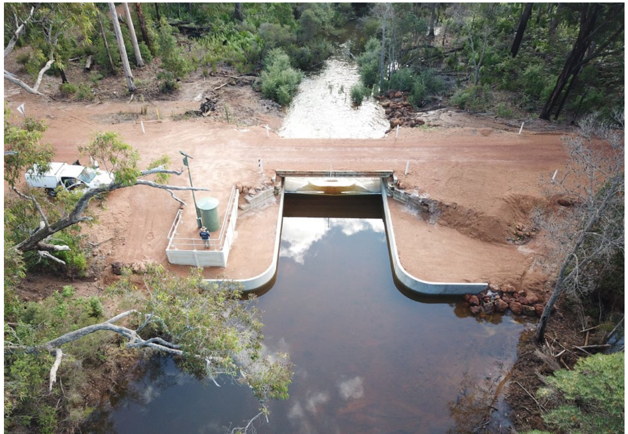
Information from gauging stations like this one at Manjimup Brook is used to develop surface water and groundwater models to assess the availability and quality of water
