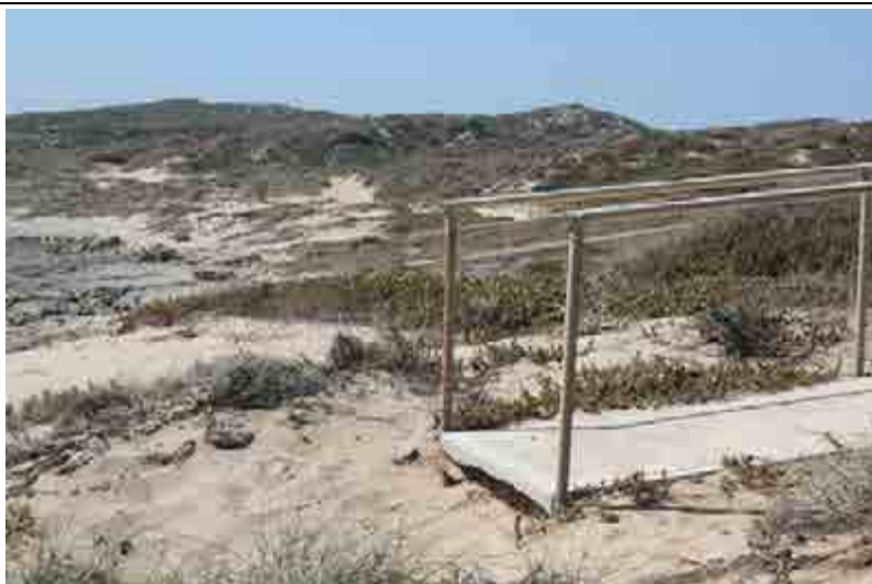
Plate 17: Erosion under access ramp
