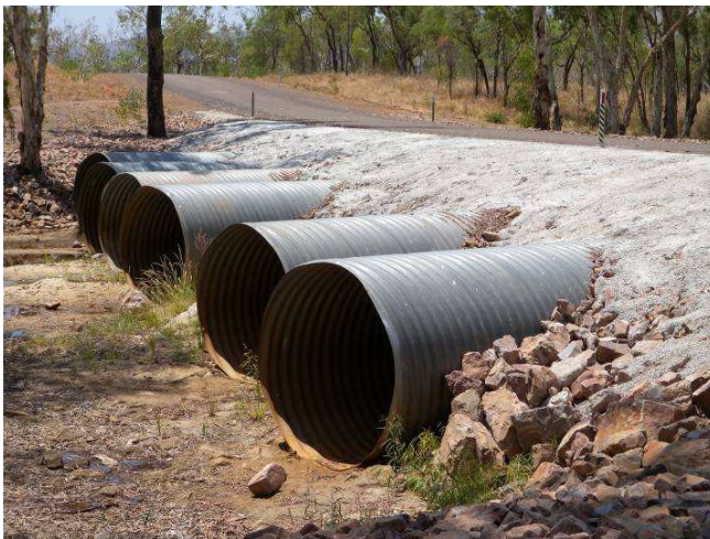
Figure 7 - Drainage culverts and causeway over Packsaddle Creek
