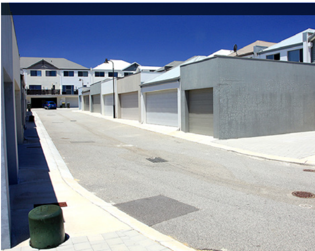
Passive surveillance of laneway
