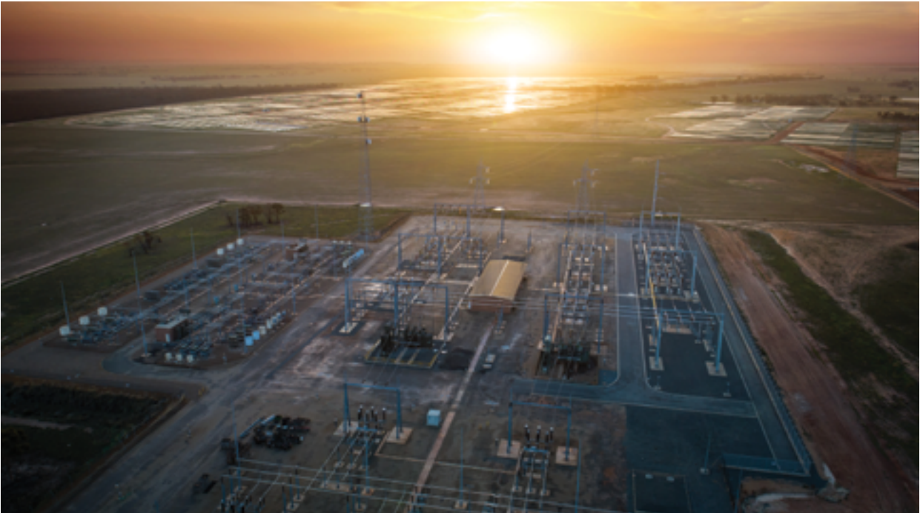
Merredin Solar Substation. Source: Western Power.
