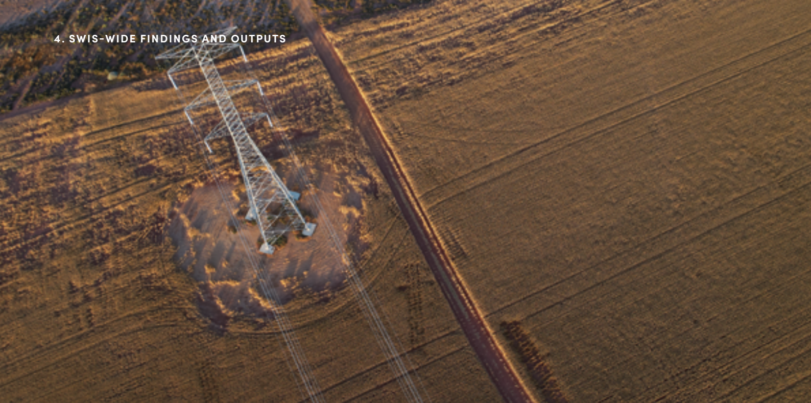
Aerial view of 330 kV transmission line. Source: Western Power.
