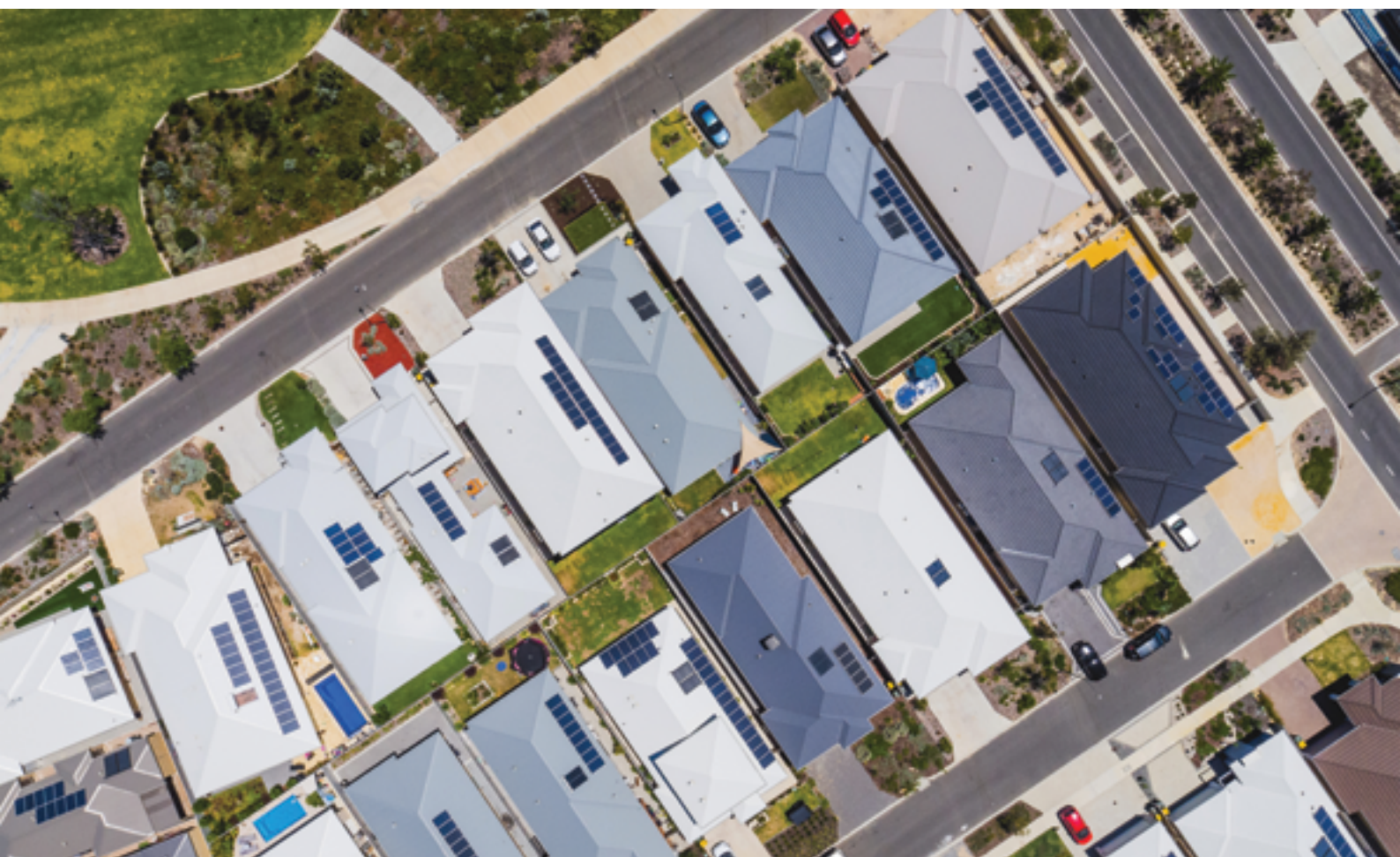
Aerial view of residential rooftop PV. Source: Synergy.
