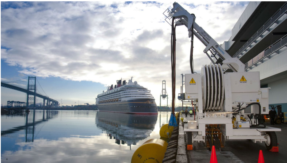
Figure 5: Cold ironing facilities at the Port of Los Angeles 31
