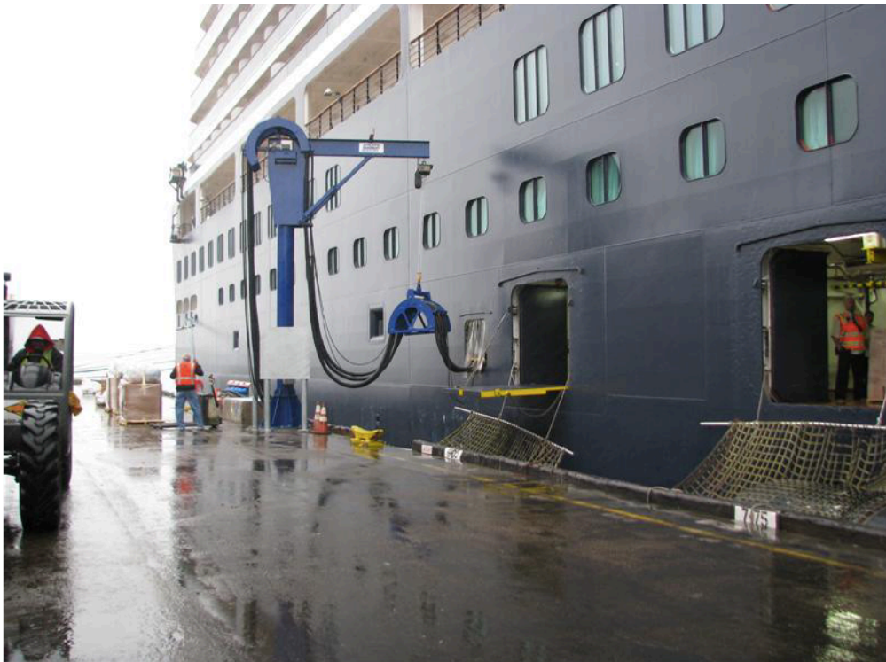
Figure 6: Cold Ironing Facilities in the Port of San Diego 34
