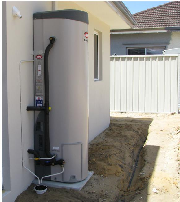
**Photo 2:** Typical insulation requirements on a storage water heater
