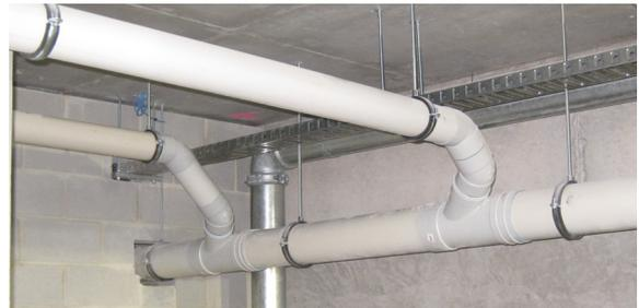
**Photo 1:** Connection of branches using unequal 45° junctions
