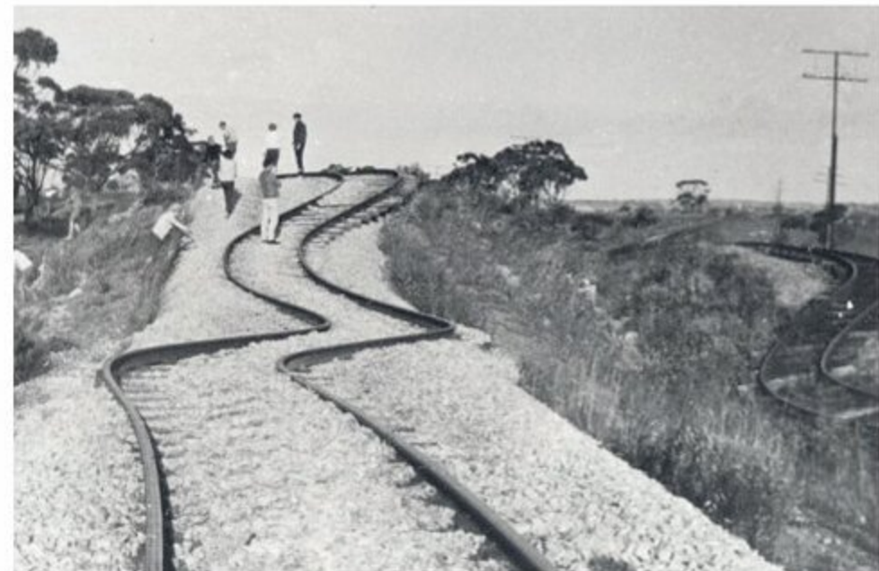
Warping of the standard and narrow gauge rail lines caused by the 1968 Meckering earthquake
